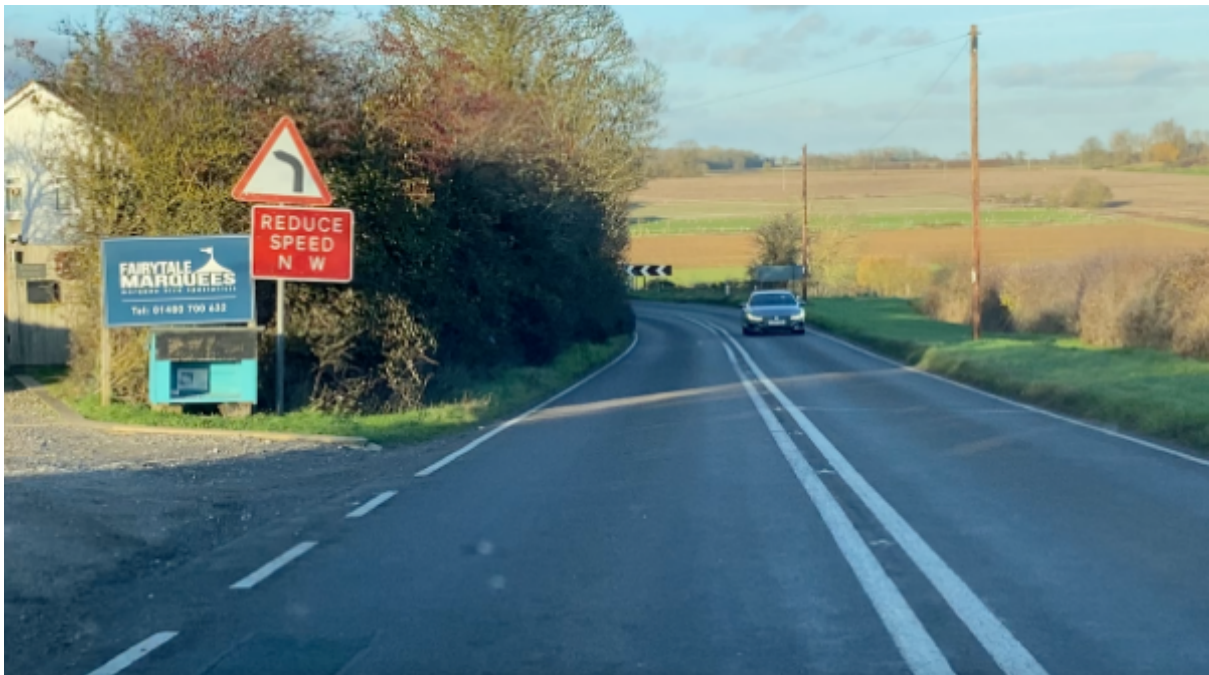
Figure S2: Downhill approach to blind left-hand bend with private access directly onto the highway.
