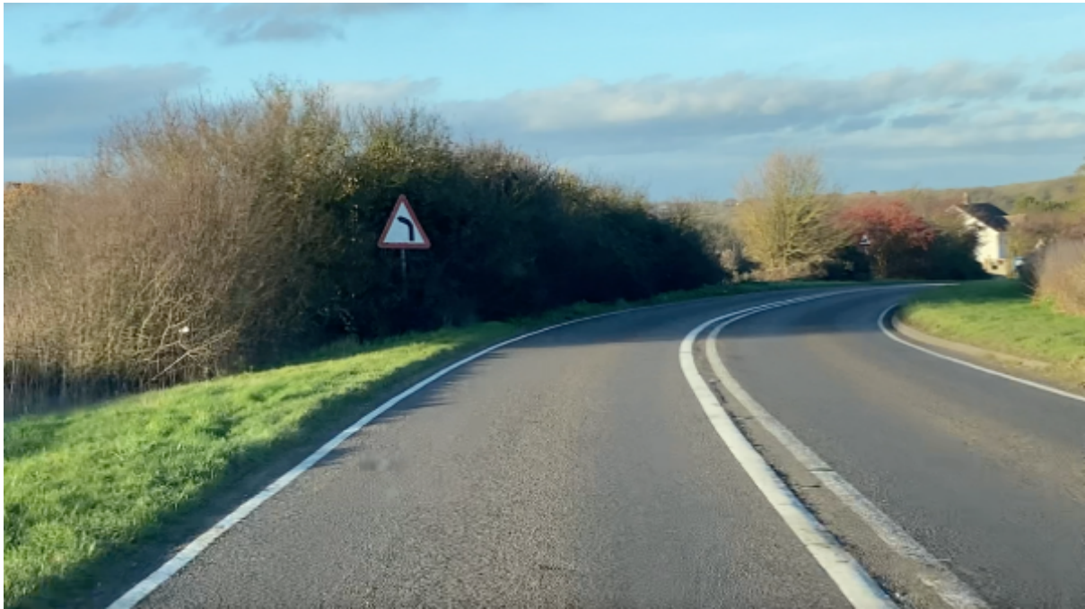
Figure S2: Downhill approach to blind left-hand bend with private access directly onto the highway.
