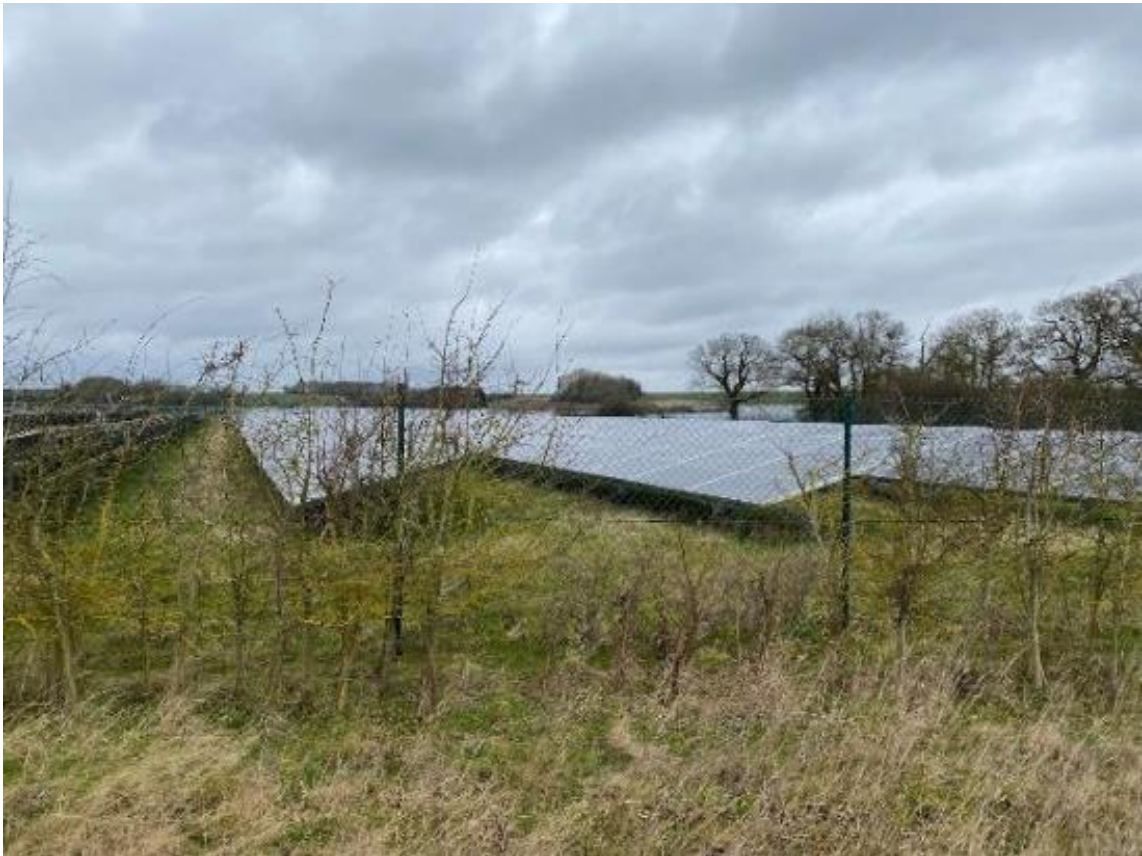
Figures G3–G4: Manor Farm Solar – ineffective screening and hedgerow failure
